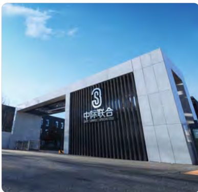
Headquarters in Beijing
